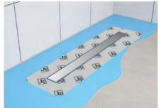
5. Unfold the membrane and slightly press it to the wet foil to ensure close adherence.
