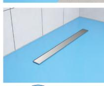
6. After drying, apply another layer of liquid foil agent onto the entrire surface, including the membrane.
