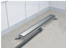
2. The adjustable legs (optional additional payment) should be glued in the places shown. Connect the channel to the drainage system and set thie height using the adjustable legs so that the upper edge of the frame is approximately 1mm below the finished surface level of the shower. We recommend that you do not remove the protective foil from the grating until the installation is complete.
